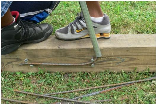
Now it time to anchor your dome to the 12' X 12' area where you have cleared the grass. You will use twenty pieces of bent rebar to anchor your dome into the ground.
